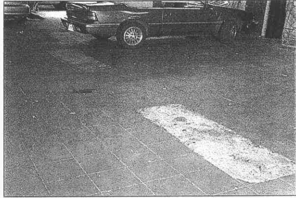
Possible location of former underground hydraulic hoists
