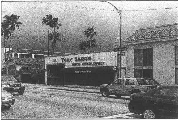
Subject property looking southeast from Colorado Street
