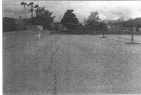
Lot 2 looking south
