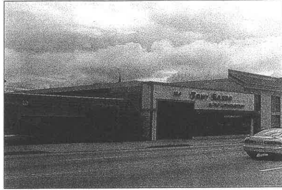
Subject property looking southwest from Colorado Street
